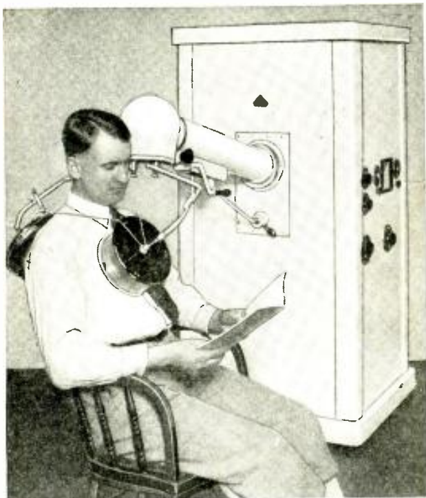
Latest German ultra-short-wave apparatus in operation. Several different types and sizes of newest ultra-short-wave electrodes with special electrodes placed on chest and back of patient.
